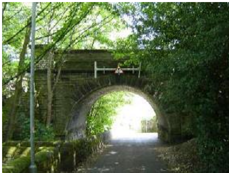
Bridge 55, Back Beck Lane Addingham
