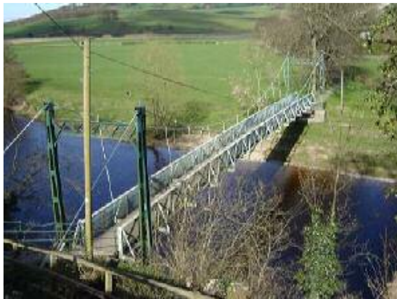
Addingham – Suspension Bridge over River Wharfe
