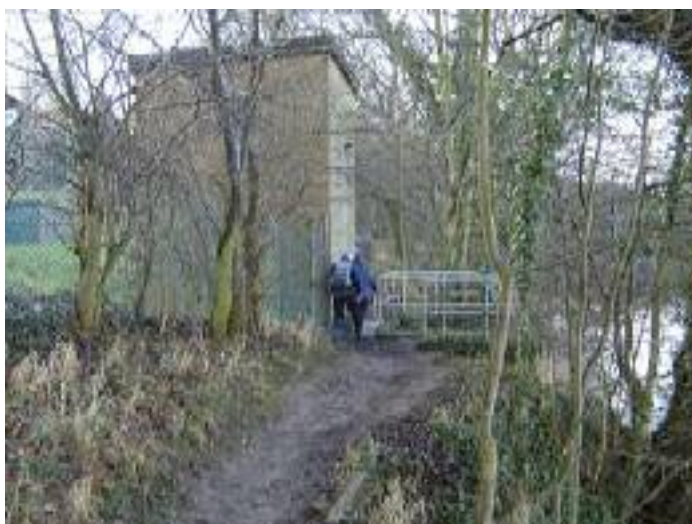
Yorkshire Water's Pumping Station near Ilkley
