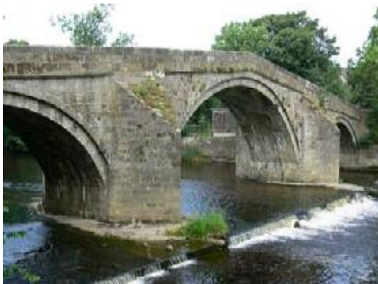
Old Bridge Ilkley
